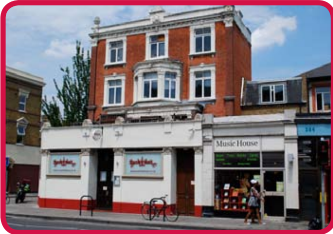
Front of Building
